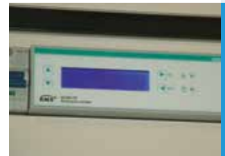
An ekinex® KNX mixing actuator controls the servo motor of a mixing valve delivering the correct temperature to the fan coil circuits
