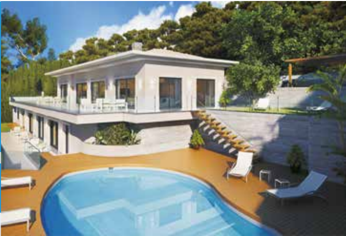
A private villa in Eze (France): complete HVAC control with KNX components, configured exclusively with ETS
