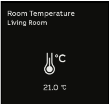
Fig. 110: Control element temperature display panel view
