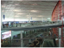
Fig.2: The world's largest airport building is equipped with KNX building control technology.
