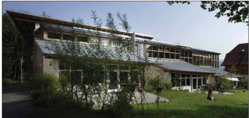
Fig. 1. The back side of the school building give an impression of the large window areas, which must be managed by the ventilation system. A weather station on the roof supplies data to the central control system.
