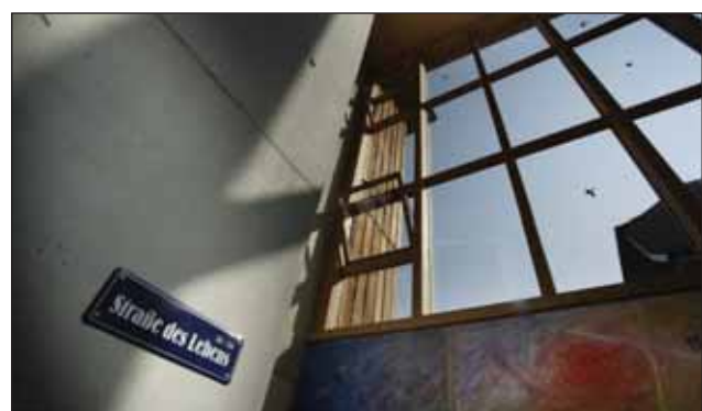
Fig. 3. Comfortable room conditions in the winter and the summer can only be maintained through an intelligent shading control system.
