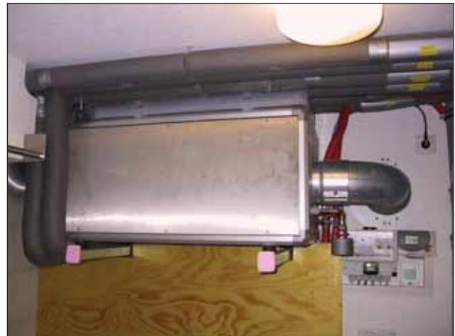
Figure 1. The air-water heat pump withdraws energy from the exhaust air stream for the heating of domestic water
