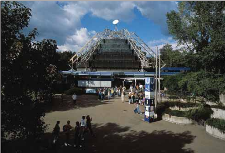
Figure 1. Planetarium Stuttgart: Straightforward retrofitting with KNX RF
