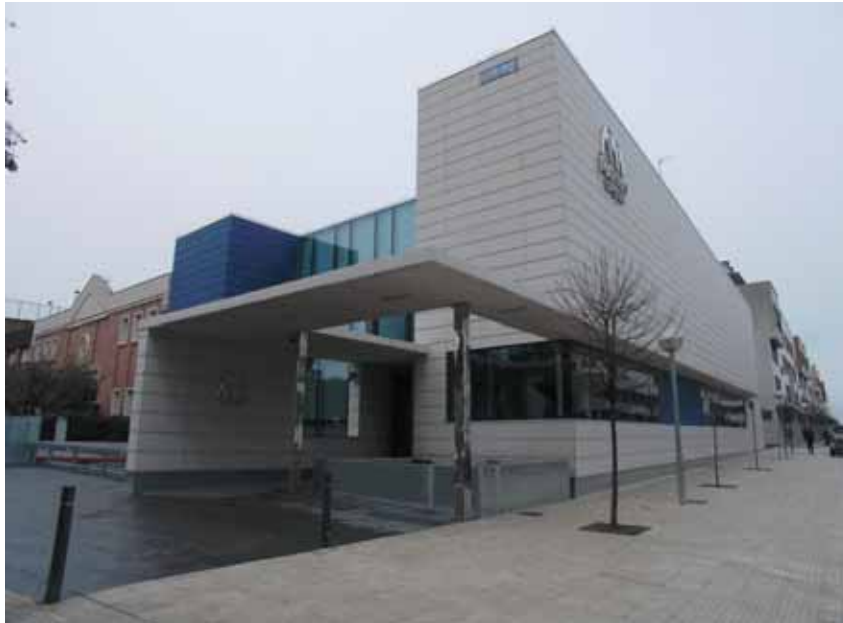
Picture 1. The new building from Marino López XXI in Huesca.
