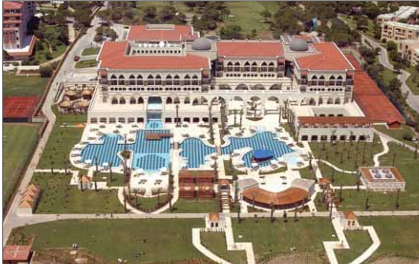
Picture 1. The Seljukian style architecture gives a special flair to Kempinski The Dome on the Turkish Riviera.
