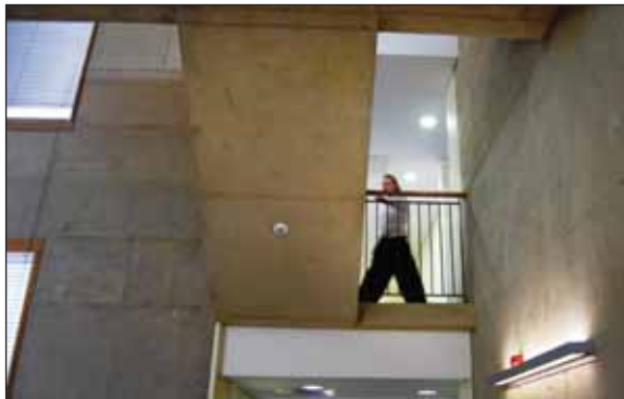
Picture 2. Energy Efficiency 2: Lots of daylight and presence sensors for the lighting system.
