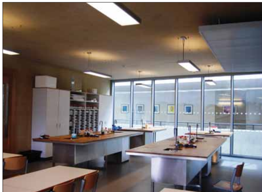
Picture 1. Energy Efficiency 1: Demand controlled lighting with KNX in the laboratories.
