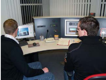
Figure 3. With the help of a visualisation showing all of the systems, fire brigade members have a reliable overview of systems and can operate them easily. Source: HTL St Pölten
