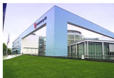
Figure 4. The headquarters of Salzburg AG, where the KNX control system for the city's street lighting was implemented. Source: Shäcke
